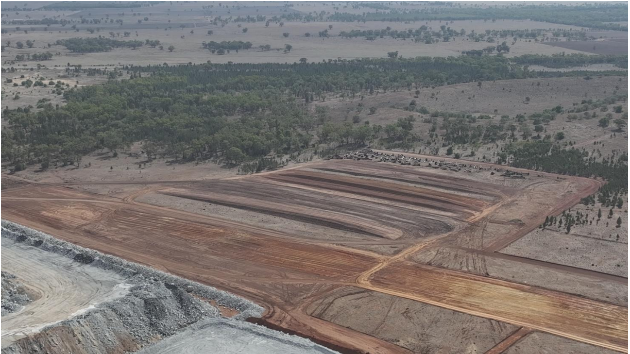
Figure 2: Image of recent clearing and soil stockpiles
